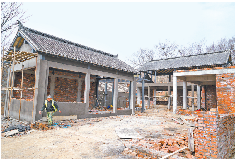
工人正抢抓工期修建民宿。⑥5
